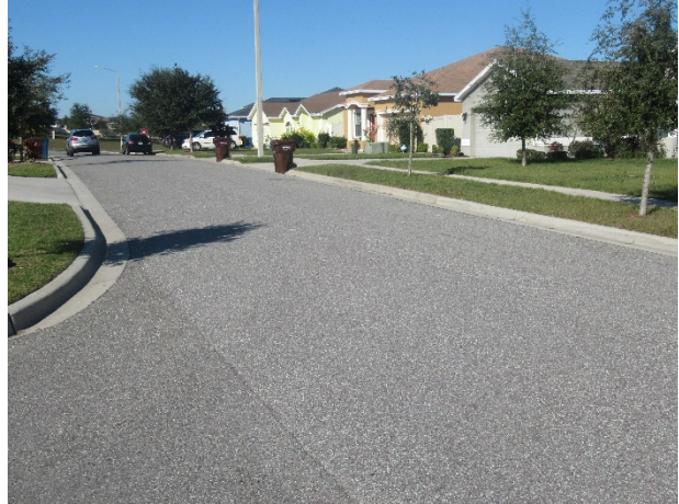
Asphalt pavement streets - overview
