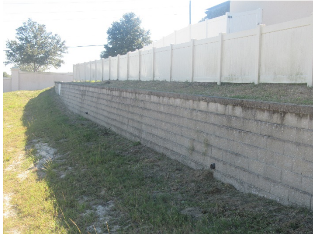
Masonry retaining walls - overview
