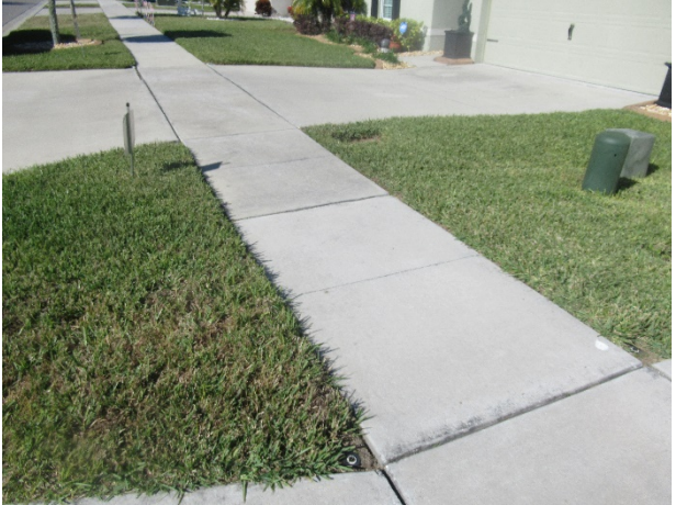
Concrete sidewalks - overview
