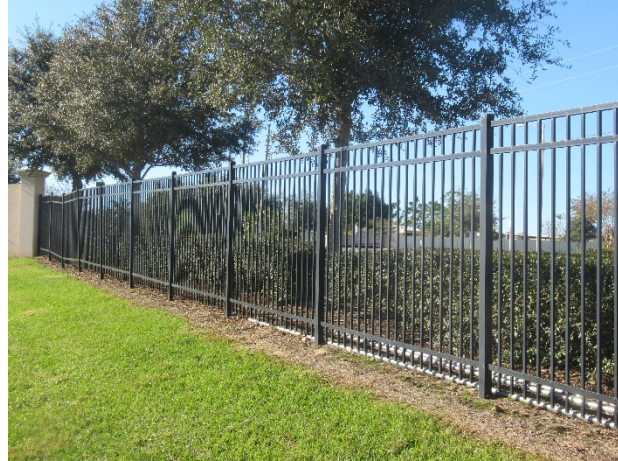
Aluminum fence - overview
