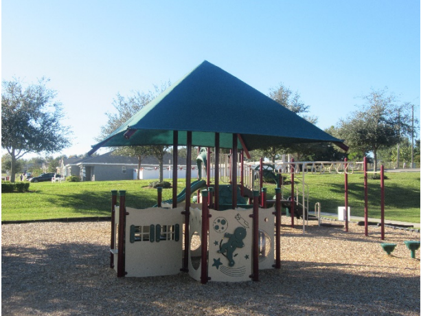
Playground equipment - overview
