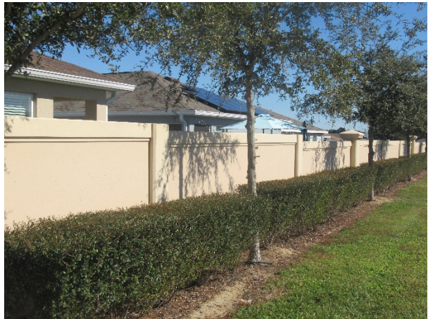
Perimeter walls - overview
