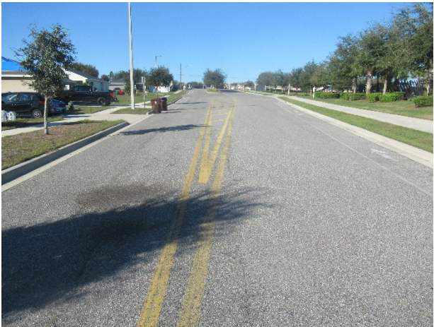
Asphalt pavement streets - overview
