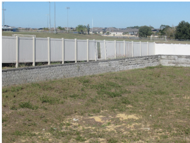
Masonry retaining walls - overview
