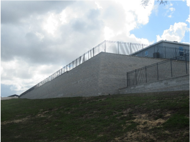
Masonry retaining walls - overview
