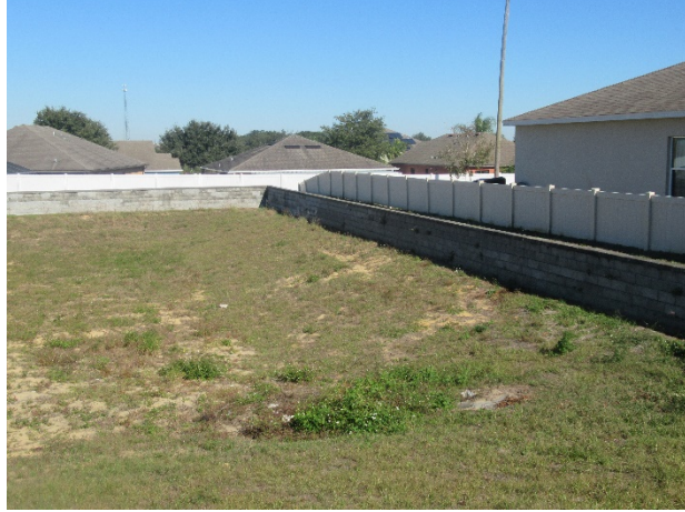
Masonry retaining walls - overview
