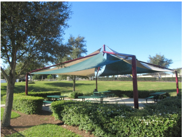
Playground equipment - overview
