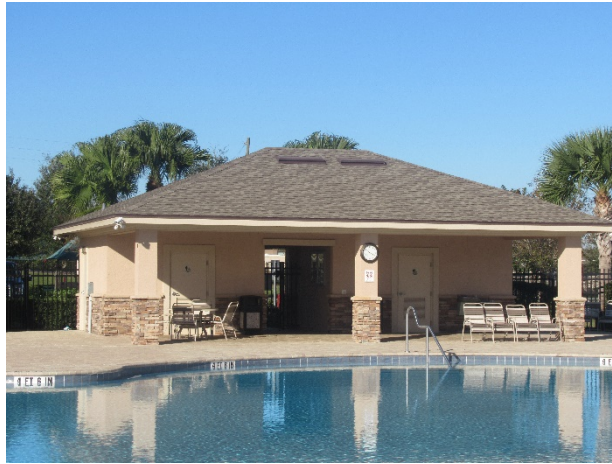
Asphalt shingle roof - overview
