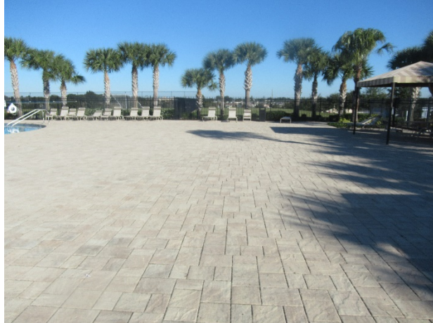
Deck pavers - overview
