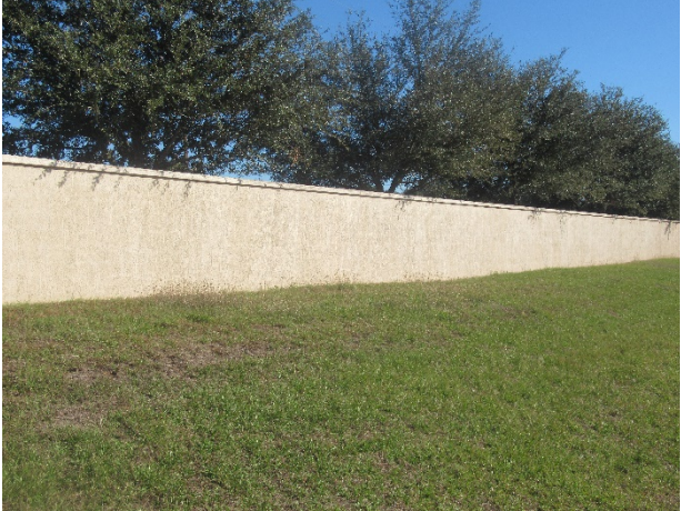
Perimeter walls - overview
