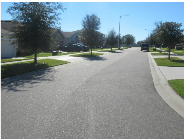
Asphalt pavement streets - overview
