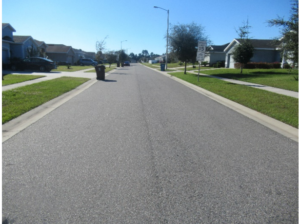
Asphalt pavement streets - overview
