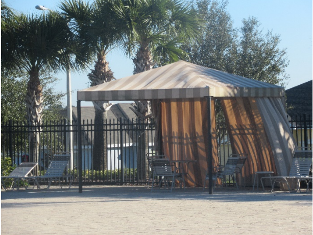
Shade structures - overview
