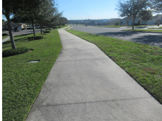
Concrete sidewalks - overview
