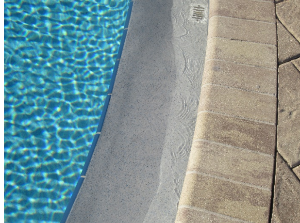
Pool finishes - overview
