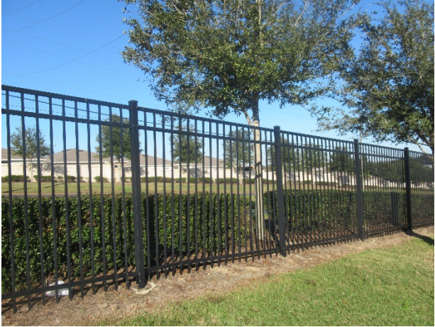
Aluminum fence - overview
