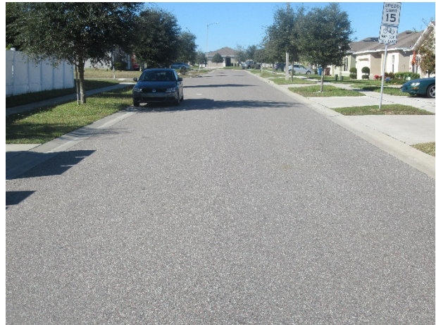
Asphalt pavement streets - overview
