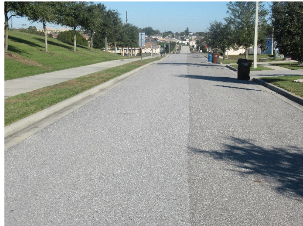
Asphalt pavement streets - overview
