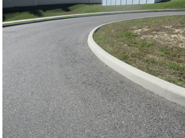
Concrete curbs and gutters - overview
