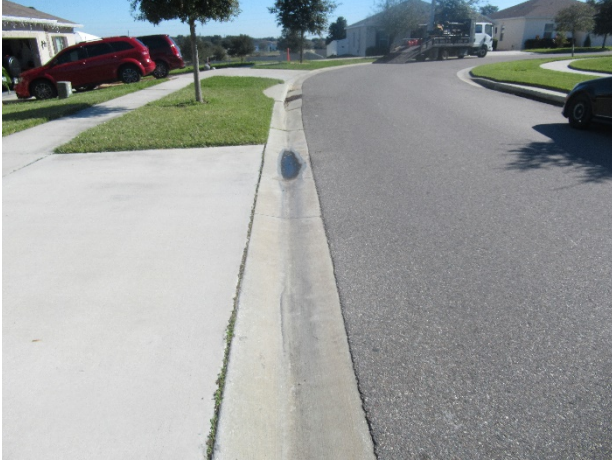
Concrete curbs and gutters - overview
