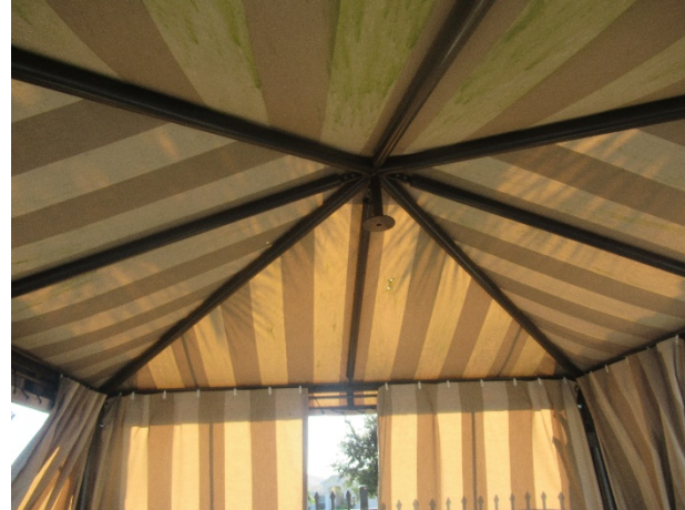
Shade structures - overview
