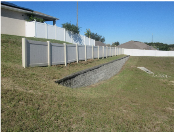
Masonry retaining walls - overview
