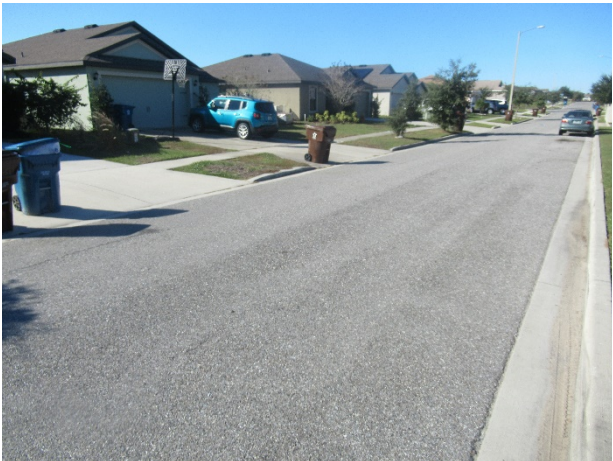
Asphalt pavement streets - overview
