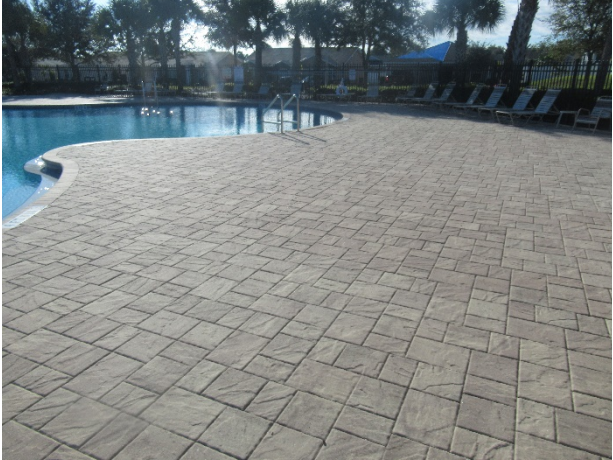
Deck pavers - overview
