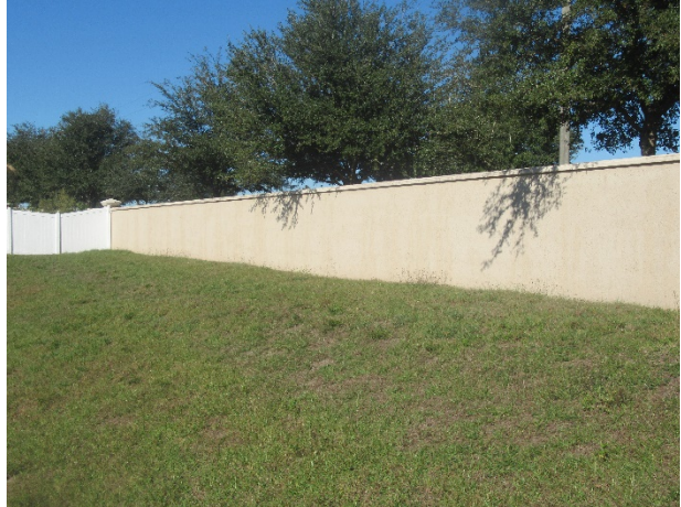
Perimeter walls - overview
