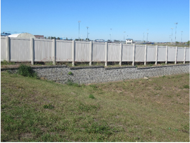
Masonry retaining walls - overview
